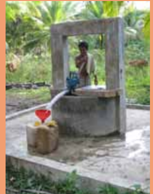
The cap, hand pump, skirting and drain channel make this well far cleaner and more efficient for all users.
