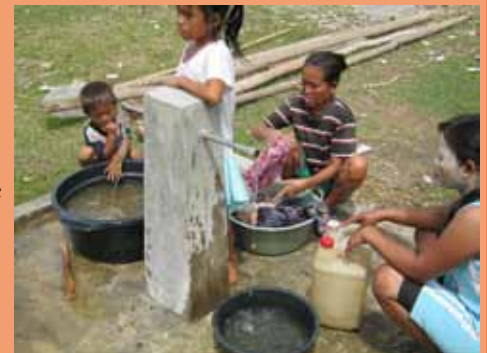
The new pump brings water from the distant pump house right into the village center.
